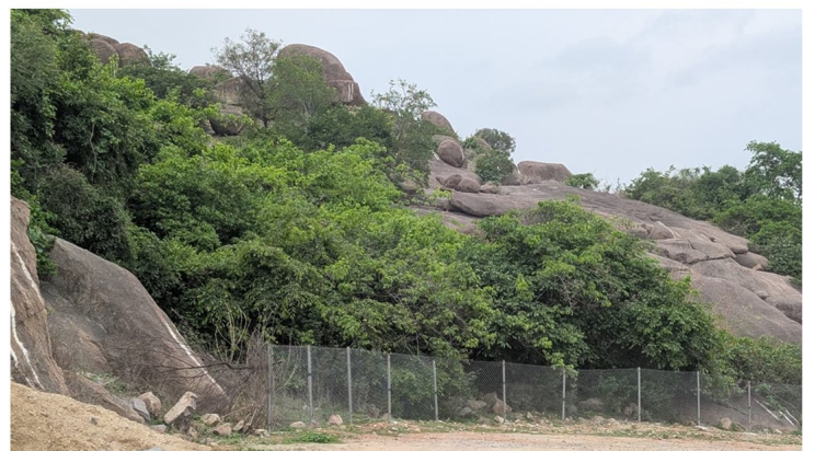
Ongoing fencing work
